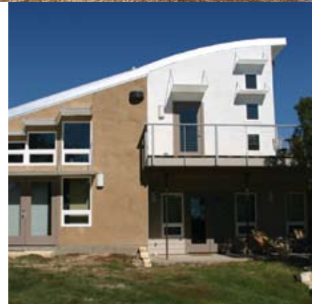
Photo courtesy of Ferrer Builders
